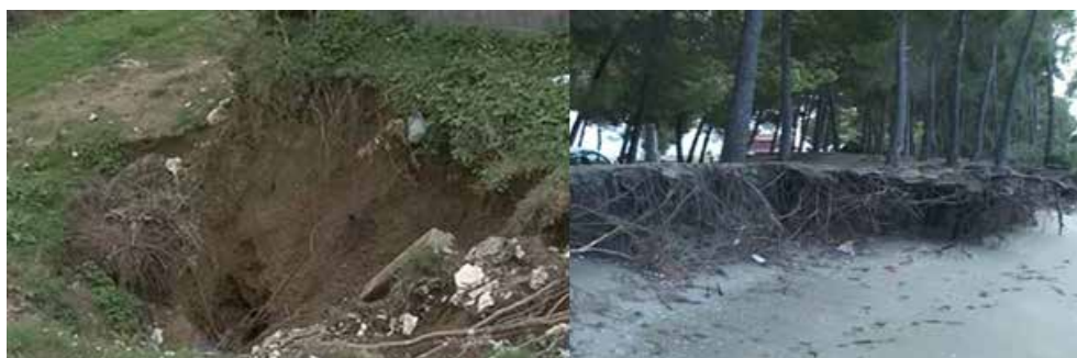
Figure 25. View from soil erosion in Albania
