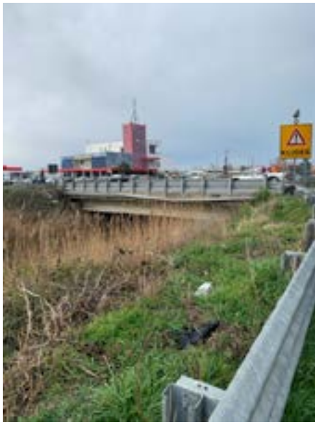
Figure 14. Photos of the Main Drainage Channel
