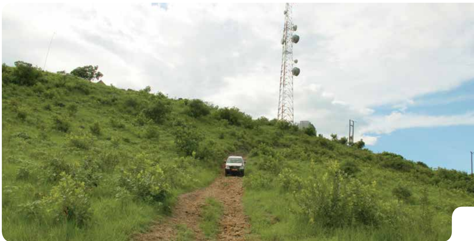
CELL TOWERS STRETCH ACROSS RURAL AFRICA, PROVIDING SECURITY, POWER AND COMMUNICATIONS FOR WEATHER MONITORING EQUIPMENT. PHOTO BY SOLOMON MANGENI.
