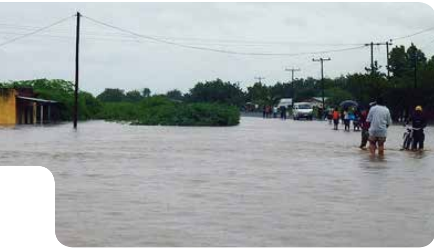
FLOODS NOT ONLY PUT LIVES AT RISK, THEY ALSO DESTROY PRODUCTIVE INFRASTRUCTURE LIKE ROADS. PHOTO BY UNDP.
