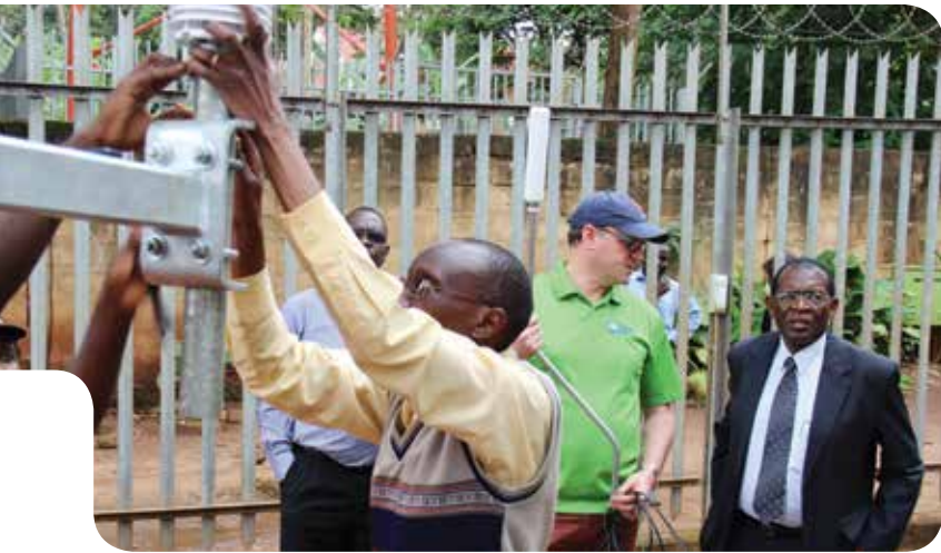
LIGHTNING DETECTION SYSTEM INSTALLATION IN UGANDA.
