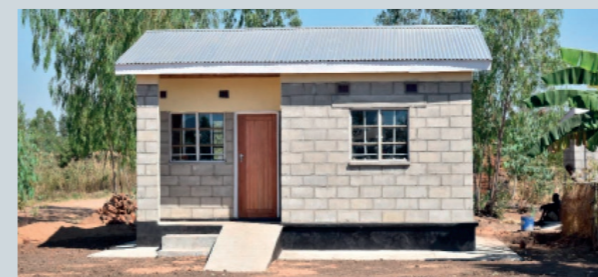
200 flood-resilient houses for the most vulnerable flood-affected communities in Malawi were constructed
