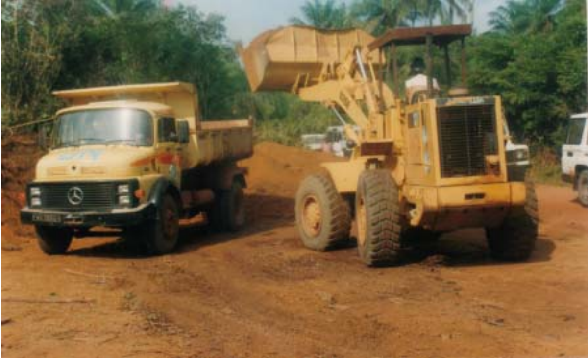
Feeder Road Construction: Working towards food security
