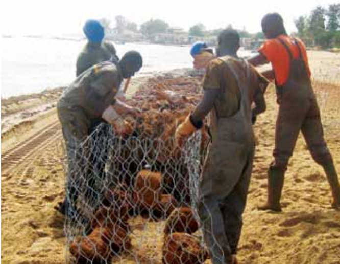
Workers in Senegal erect a rock-wall to prevent coastal erosion along a lucrative stretch of tourist-friendly coast. Supported by the AAP, this project helped the country protect a key source of revenue and identified an approach that is now being replicated elsewhere.
