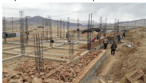
Figure 2: Construction of Nili CSC, Daikundi resumed
