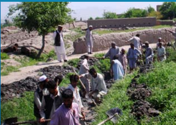
In Jalalabad, canal clearing work.
