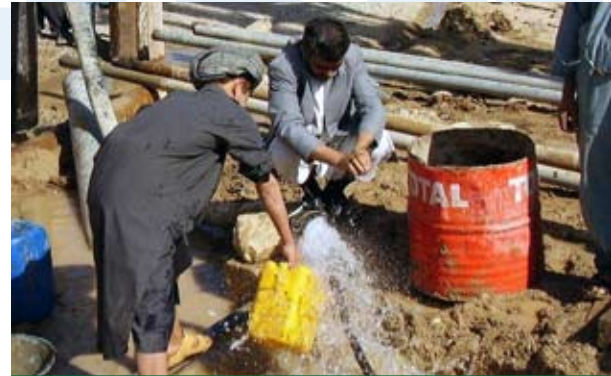
Water-well project, Samangan.
