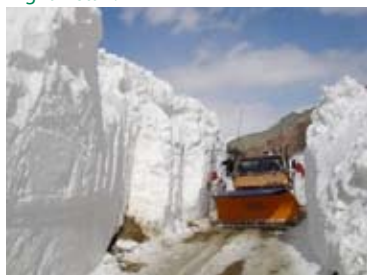
Snow clearance to open roads, southeast Afghanistan.
