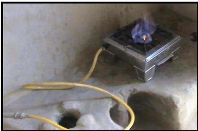
Figure 4: Completed Biogas Project in Kama District, Nangarhar Province (Photo Credit: Mohammad Asghar)
