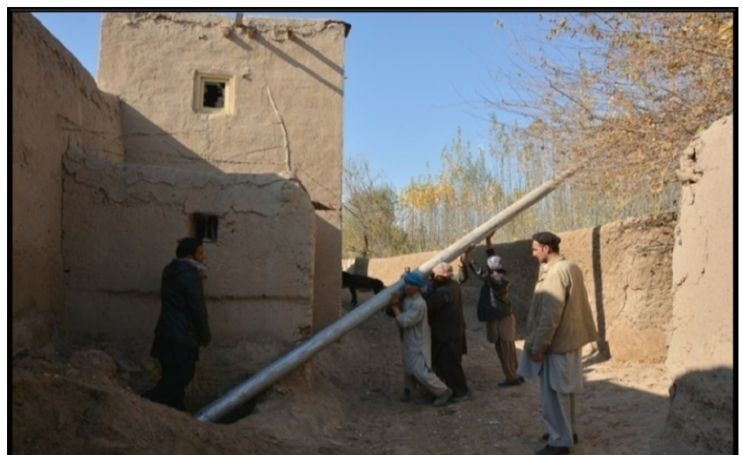
Running Pipes for an MHP Plant | Balkh Province
