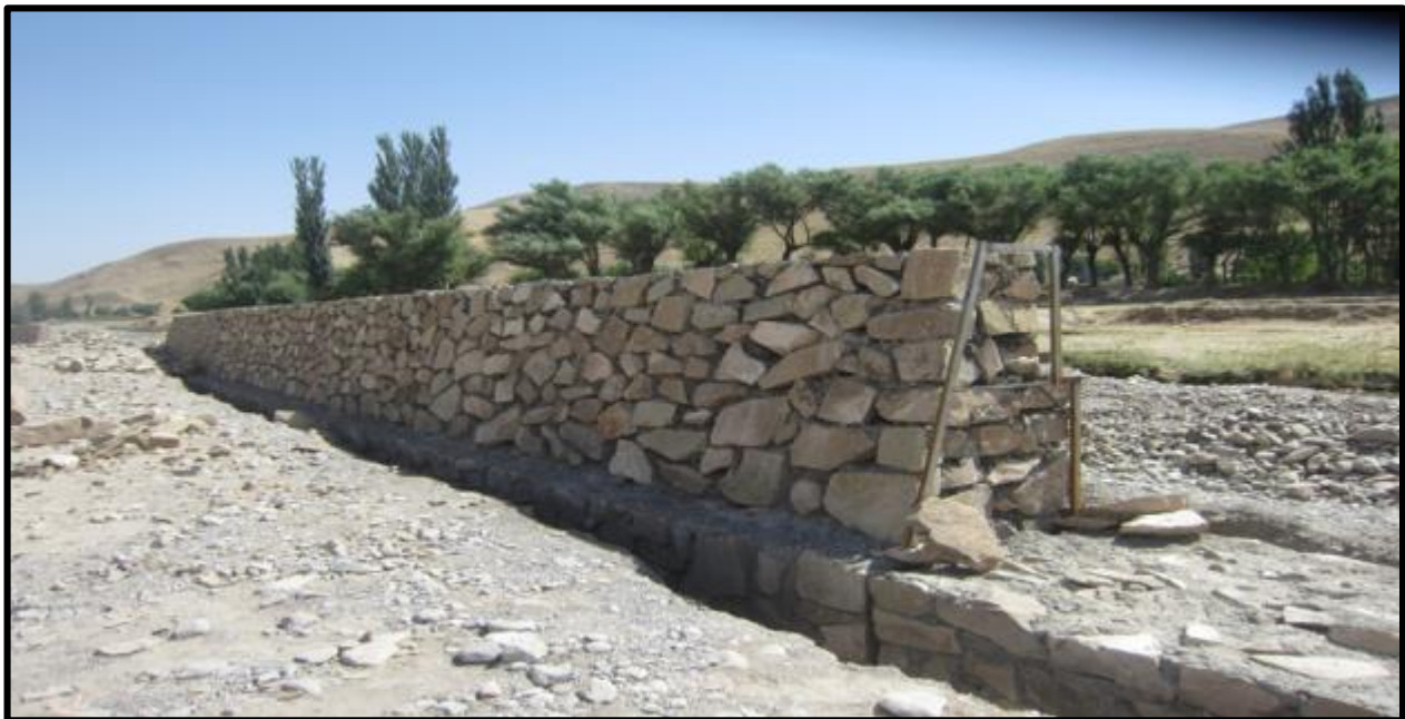
Construction of Protection Walls for the Wells
