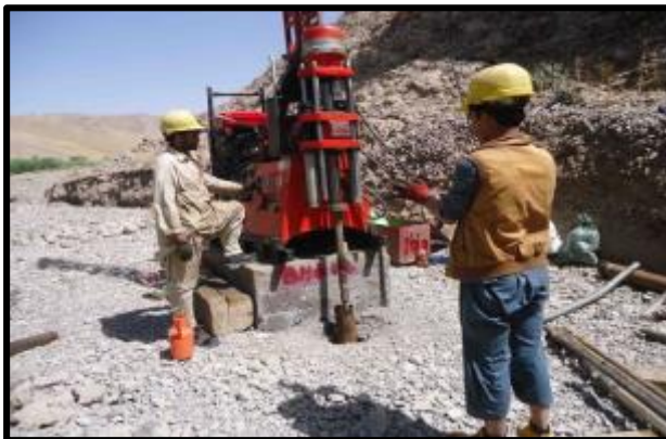
Work in Progress drilling of the Dam Site
