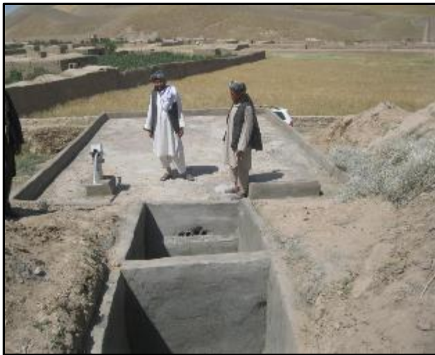
Water Reservoir Project | Muqur district | Badghis Province | Photo credit: NABDP © 2015
