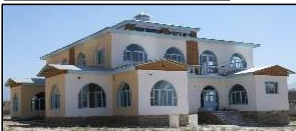
RTP Administrative Building | Deh Sabz district | Kabul Province | Photo credit: NABDP © 2015
