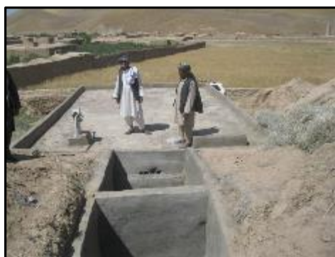
Water Reservoir Project |Muqur district| Badghis province| Photo credit: NABDP © 2015
