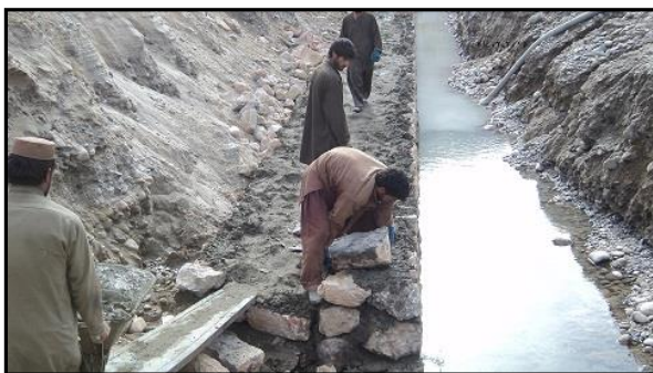
Protection Wall Project | Gizab District | Uruzgan Province | Photo credit: NABDP © 2015
