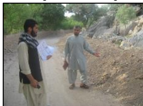
Evidence of PMT | Road Gravelling | Anar Dara District | Herat Province Photo credit: NABDP © 2015
