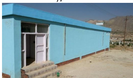
Figure 2: Construction progress Daikundi CSC
