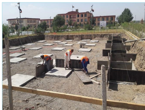
Figure 1: Ongoing construction – Khost CSC
