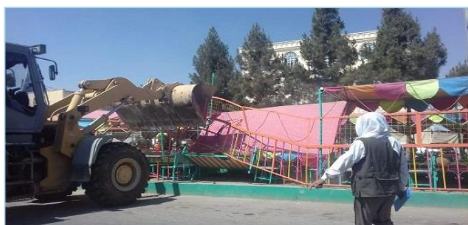
Figure 7: Demolition of illegal shops in Balkh Province
