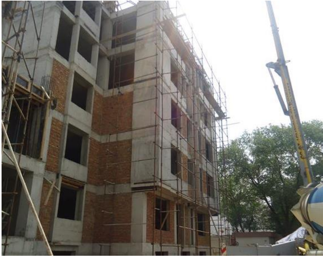
Picture 1: View of the DM Support building. Source: LOTFA.
