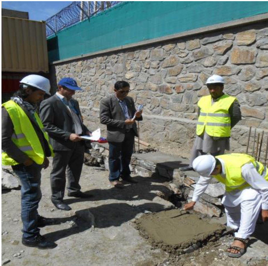
Picture 2: On-going works for women toilets construction. Source: LOTFA.
