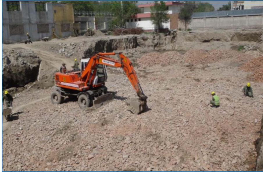
Photo 3: DM for Administration Building project. Workers cover the foundation area with mountain rocks to strengthen the overall building structure. Credit: Mol.
