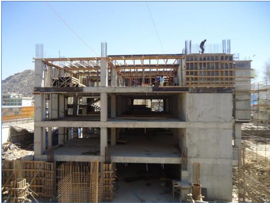
Photo 1: Construction progress at the DM Support building project site. Source: LOTFA.
