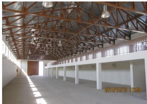
IEC warehouse in Herat. Photo: ELECT II.
