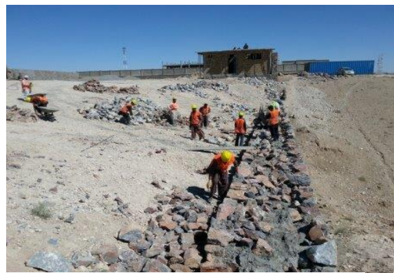
Boundary wall at Zabul
