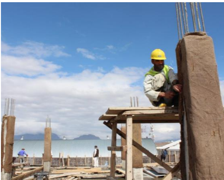
Construction of the IEC Training Centre
