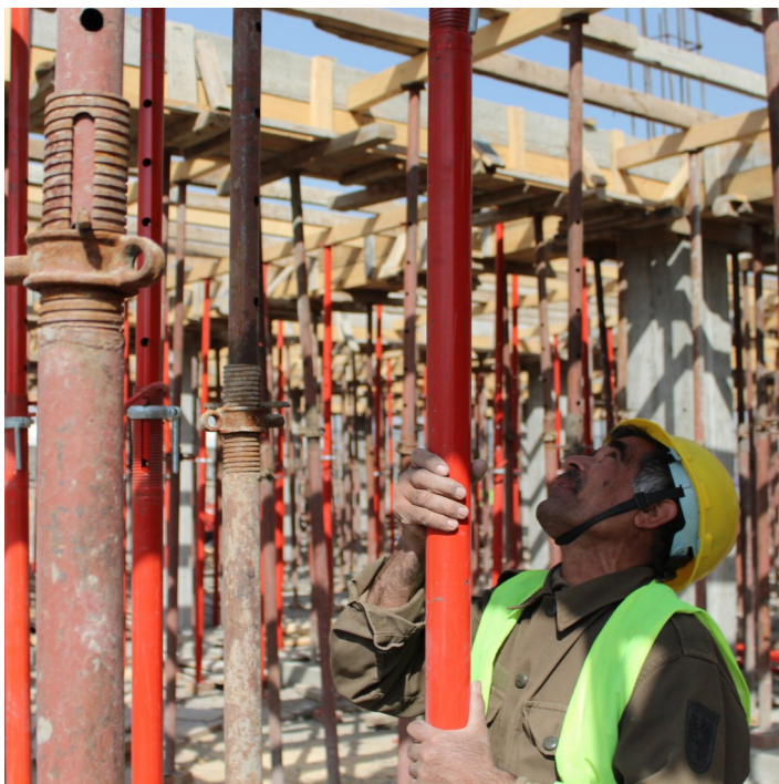
IEC's Training Center construction
