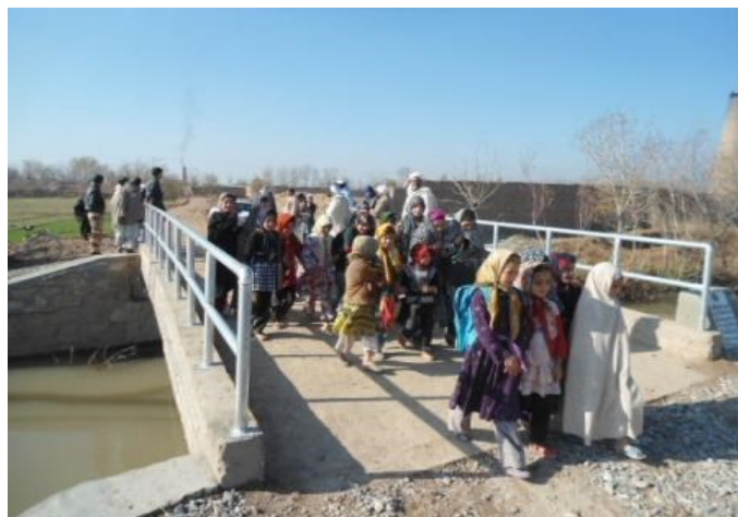
Connecting communities in Herat. Bridge built with SGP funds
