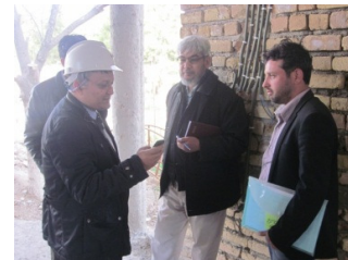
Monitoring of Customer Service Centre Construction (Photo credit: ASGP)
