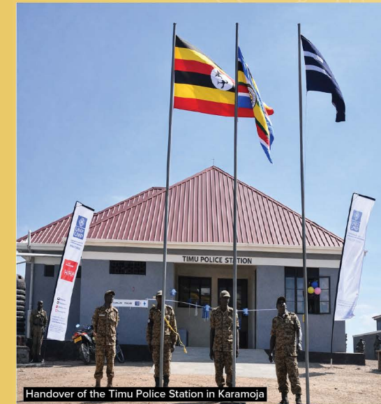
Handover of the Timu Police Station in Karamoja
