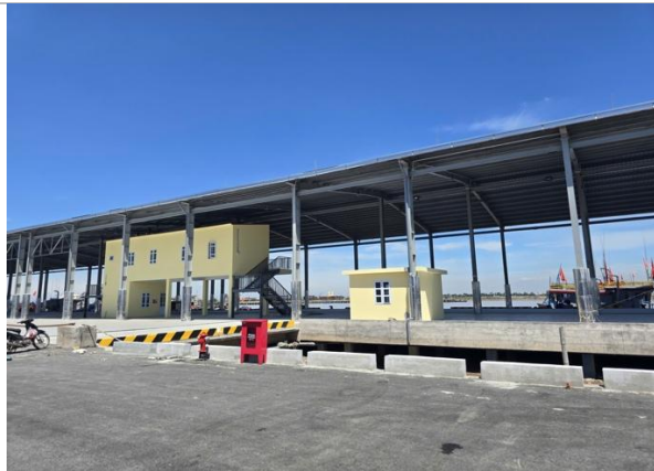
Picture 11. Fire prevention and protection system in Ninh Co Fishing Port
