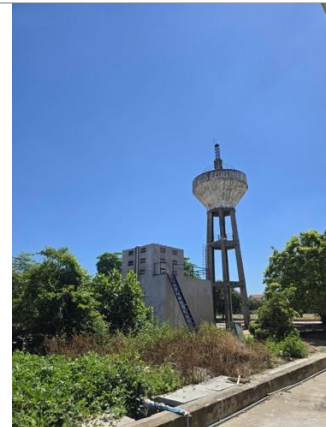
Picture 12. Fire prevention and protection system in Ninh Co Fishing Port
