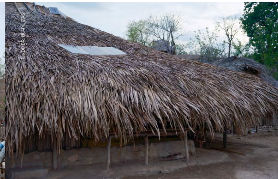
A glimpse of how the solar panels are installed on traditional homes in the village of Uma Naruc
