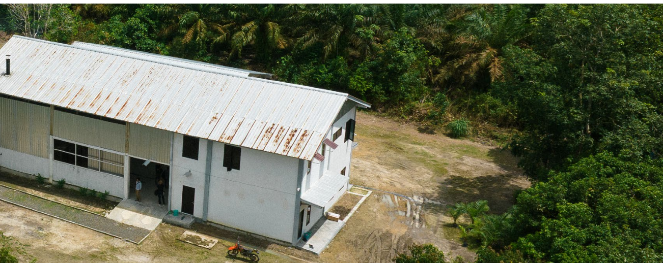
Product Development Center (PDC) in Seruyan that houses nursery, processing, and research facilities for patchouli under the Gawi Bapakat initiative.
