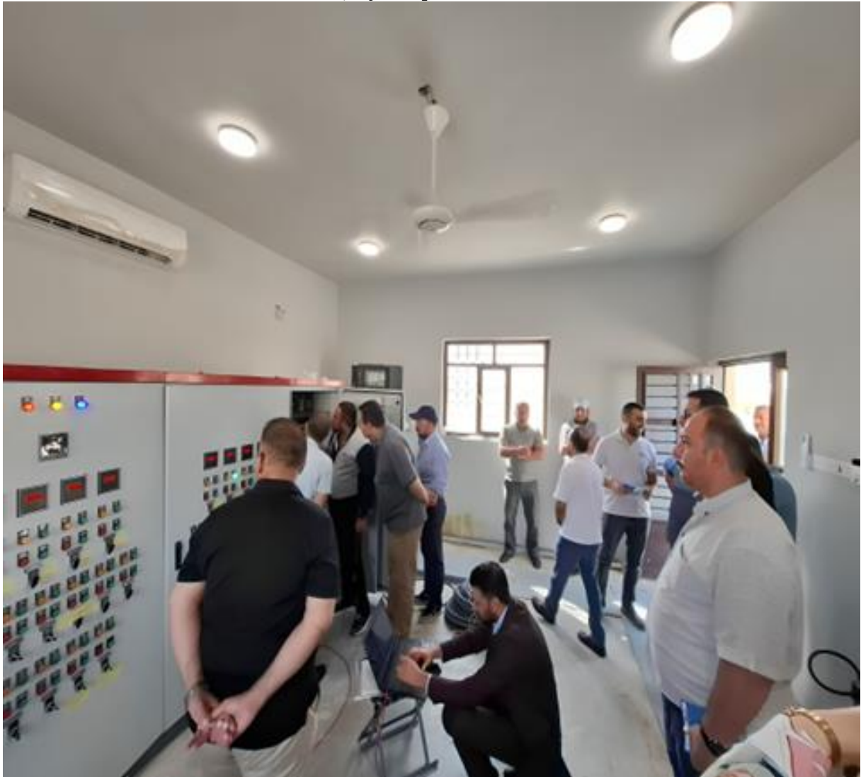
Sewerage employees testing a SCADA system on Baiji Sewerage Plant, September 2024. (photo credit, UNDP Iraq)
