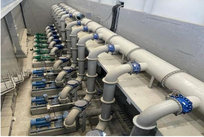
REHABILITATED STORMWATER LIFT STATION PHASE 2, JUBAIL DISTRICT, FALLUJAH, SEPTEMBER 2024
