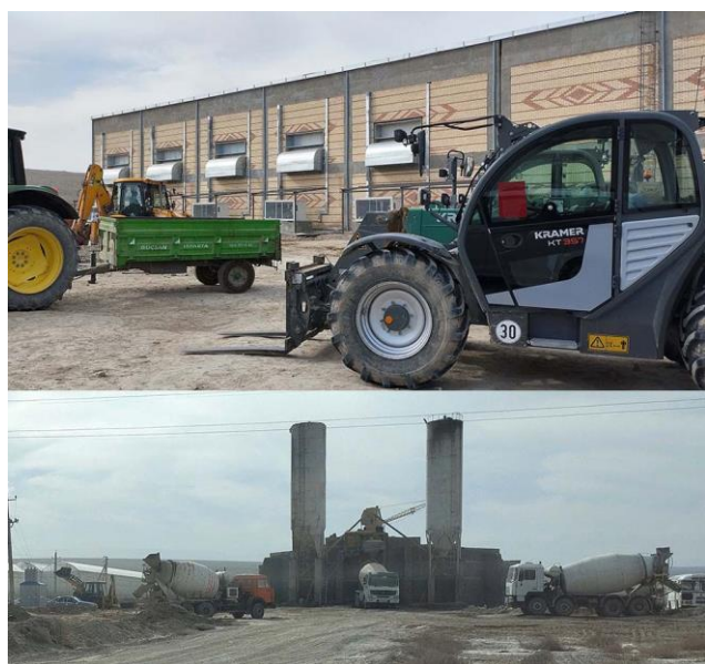
Photo 4. Construction of new industrial refrigerators for storing of grown products
