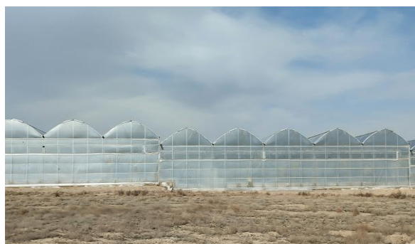
Photo 7. Banana greenhouses (exterior view)
