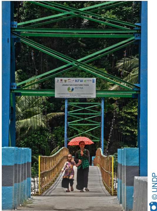
The suspension bridge of Tuva Village connects the community to their resources, which sustain their economic and livelihood activities.
