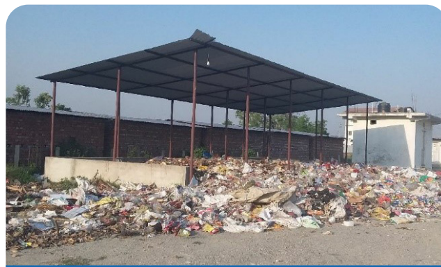
Figure 2-5 Solid Waste Management facility at Duhabi Municipality (Source: Authors)
