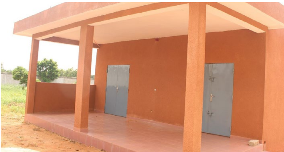
Shelter for implementing explosives
