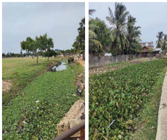
Figure 6-5: Thona in the city Clogged up Aquatic weed Eichonia crusipae (Japan jabara/water hyacinth)
