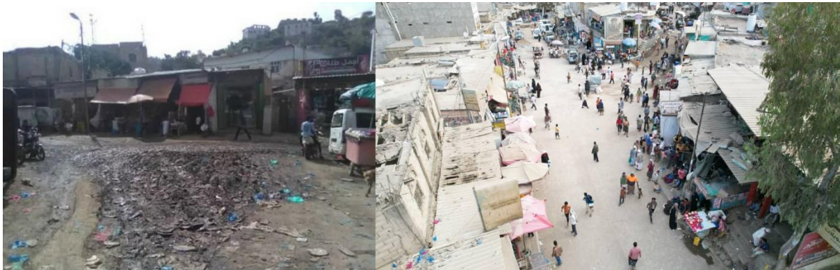
Al-Nashamah market before and after rehabilitation, Al-Ma'fer district, Taizz.
