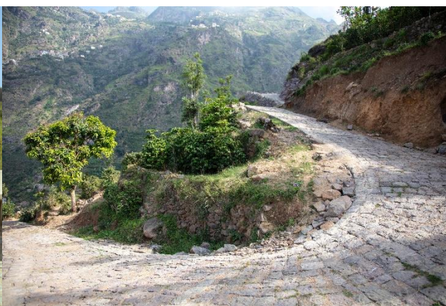
Al-Maghrabah road rehabilitation in Milhan, Mahweet
