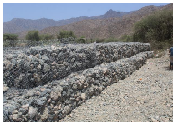
A constructed gabion wall in Lawdar, Abyan
