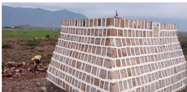
Water tank built in Bajil, Hudaydah
