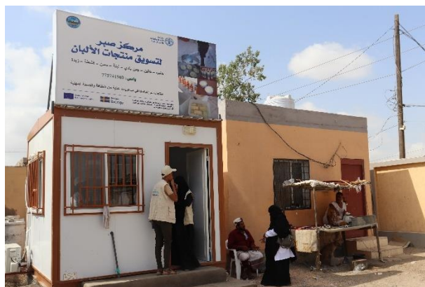
Installed dairy marketing center in Saber, Lahj Governorate.
