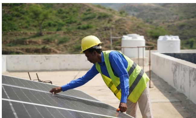
Installation of Solar Systems in the Alzahra school, Najrah District.
