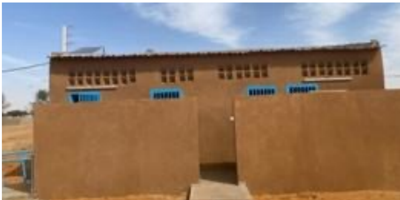
Construction of public toilets, Seytenga © UNDP Burkina Faso
