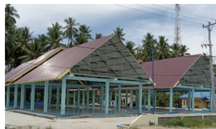
The Omu Market after reconstruction. The market was damaged due to the earthquake in Palu in 2018. Credit: UNDP Indonesia – PETRA Project.
