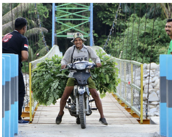
A local resident in Tuva Village crossing the bridge after being renovated. The two villages were disconnected due to the damaged bridge during earthquake in Palu in 2018 Credit: UNDP Indonesia – PETRA Project.
