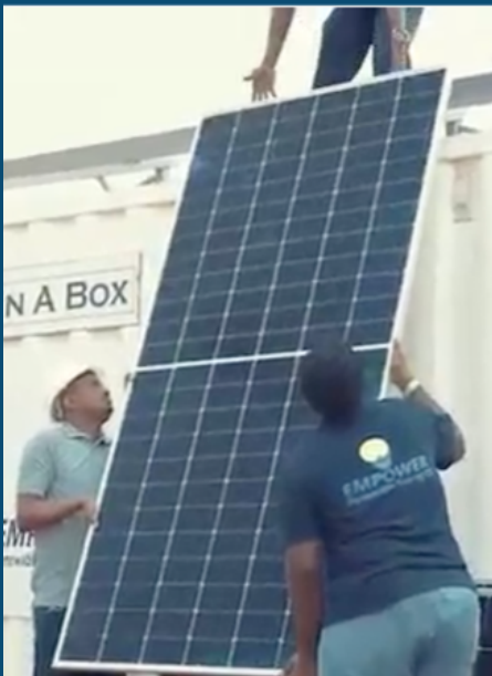
Constructing a Solar-in-a-Box unit. Image: Empower Energy Service Company.
