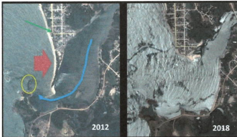
Figure 14. Satellite photos of the Sinoe River delta in Greenville taken in February 2012 (left) and March 2018 (right) show sizable erosion of the Greenville peninsula area resulting in more than 50 houses being eroded or incapable of further habitation (red arrow). In addition, the southern tip of the main Mississippi Street and side streets (green arrow) have been completely eroded. The blue arrow represents the main river current direction along the original riverbed. A shipwreck (from 1990s civil war) at the mouth of Sinoe River delta has been encircled yellow and is believed to possibly have a function in redirecting local ocean bay currents towards the Mississippi Street area, which will be exacerbated by projected climate changes including an increased frequency of high-intensity rainfall events 184 .
