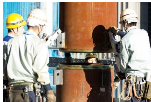
Scene on site
