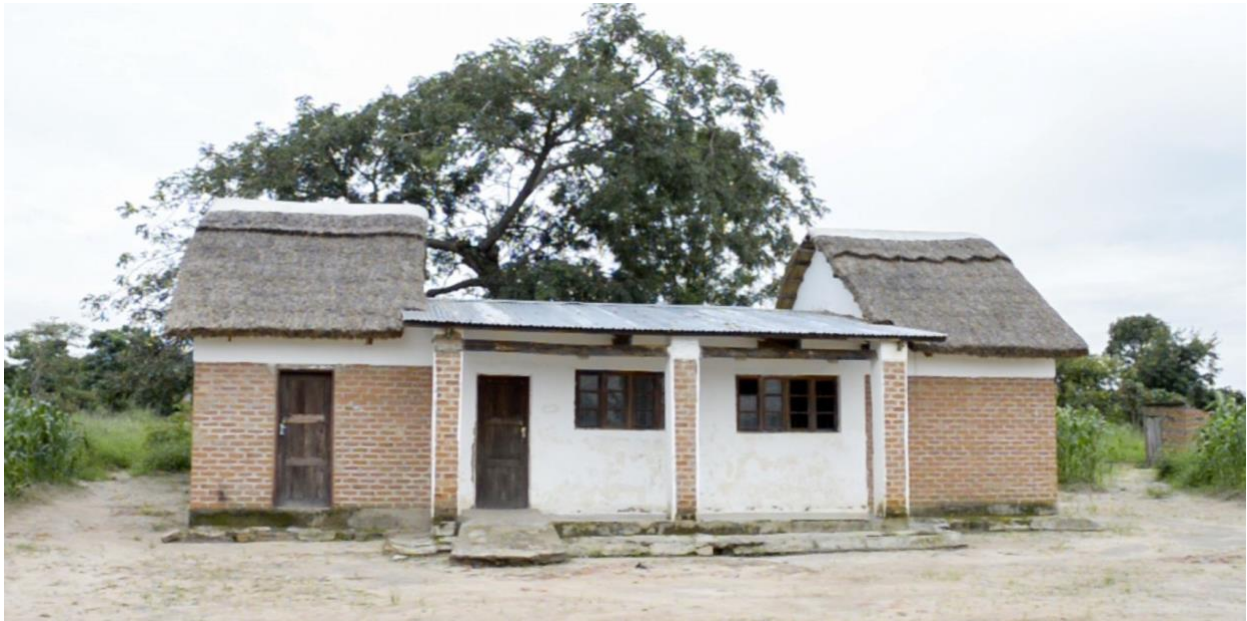
Figure 6: Improved aggregation and storage centre
