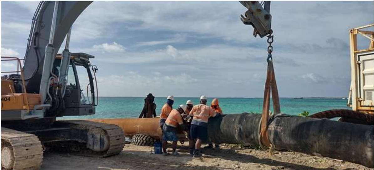
Figure 15: Dredge pipeline being moved on shore. Photo credit: P.Hawes
