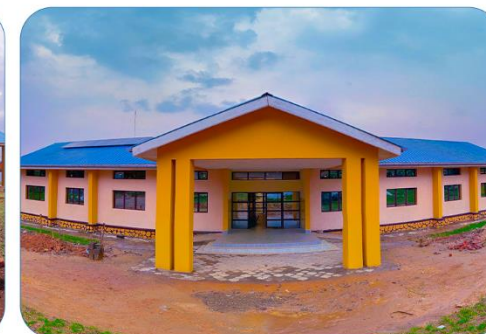
BATIMENT ADM IDJWI-TERR IDJWI
