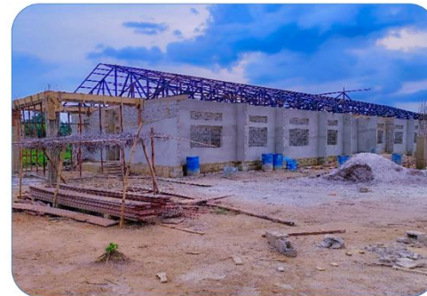
BATIMENT AD BEFALE CENTRE -TERR BEFALE
