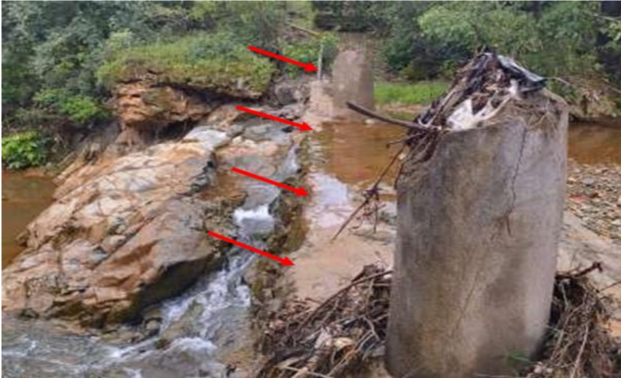
Plate 4: Delivery pipeline buried in Concrete, at Shekani River Crossing
