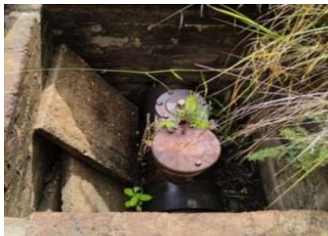
Plate 3: Air release valve on 300mm Dia Section
