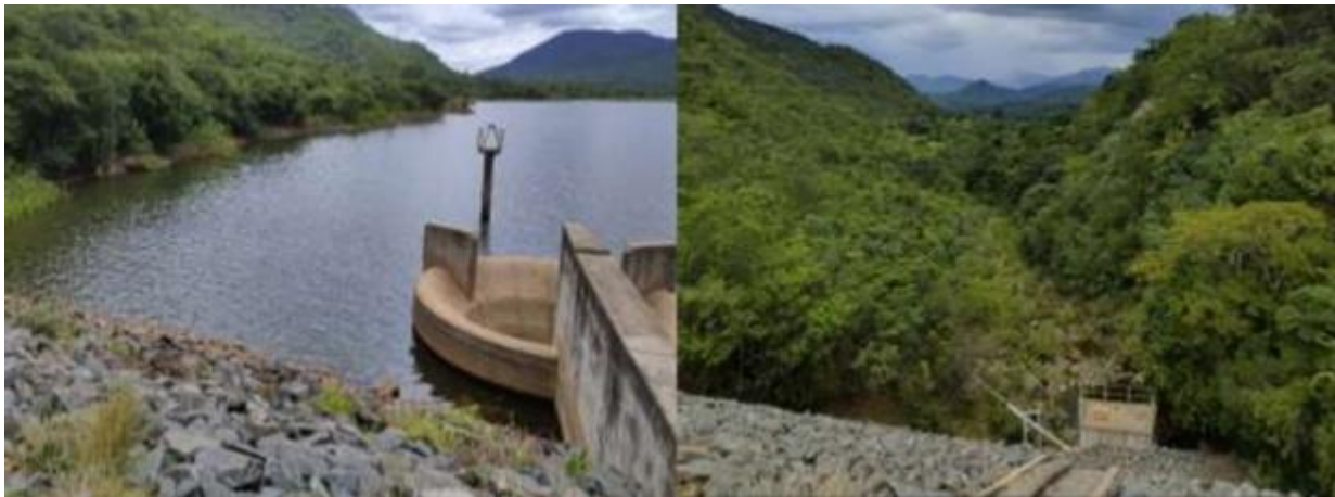
Plate 1 Dam Spillway and Outlet Pipe
