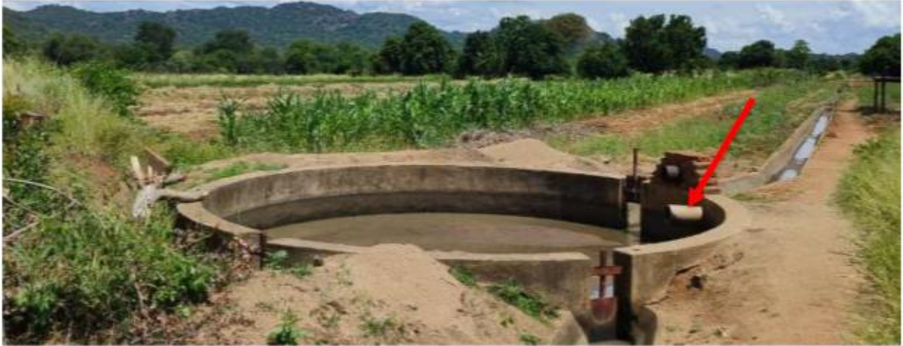
Plate 13 Distribution Chamber with 3 sluice gates connected to canals
