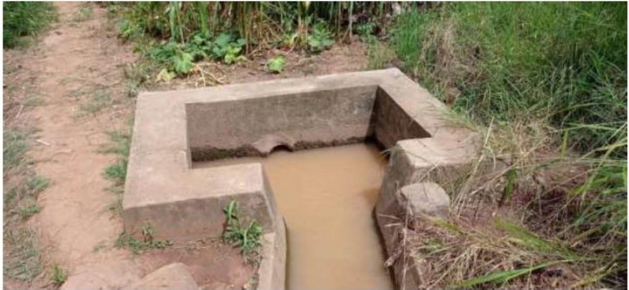
Plate 9: Outlet from the weir into the main canal
