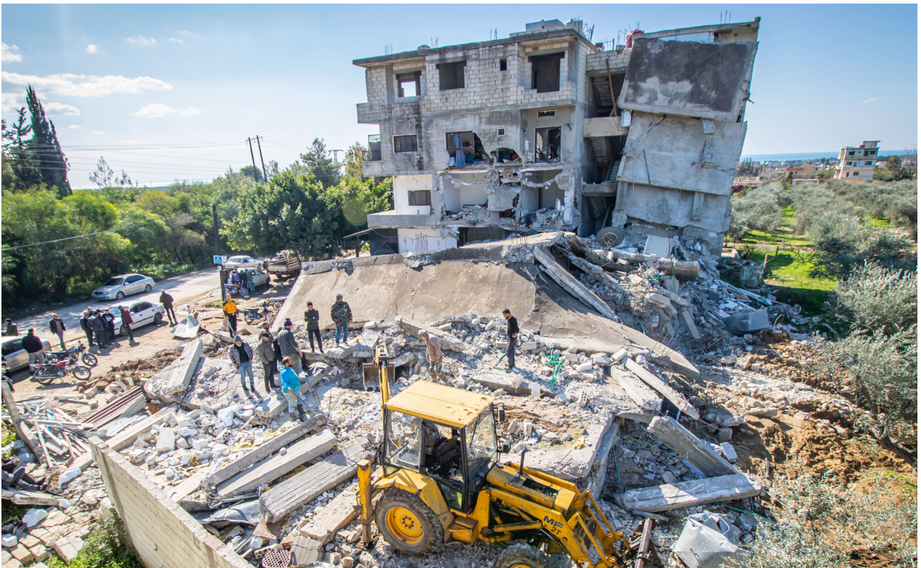
Image displaying damage post earthquake catastrophe
