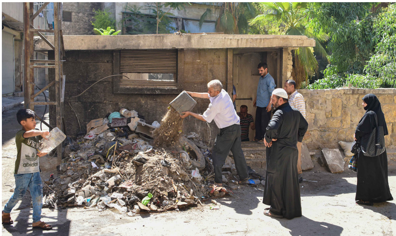
Figure 3.2. Local community initiative - rehabilitat electrical transformation building
