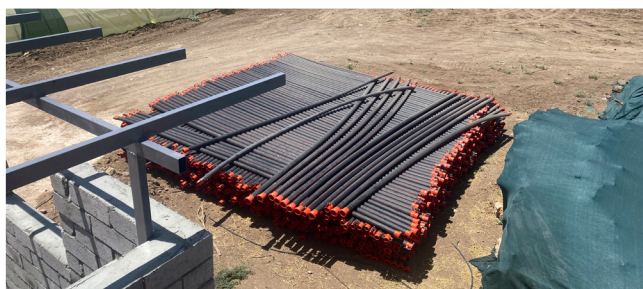
Green House in Bashiqa
