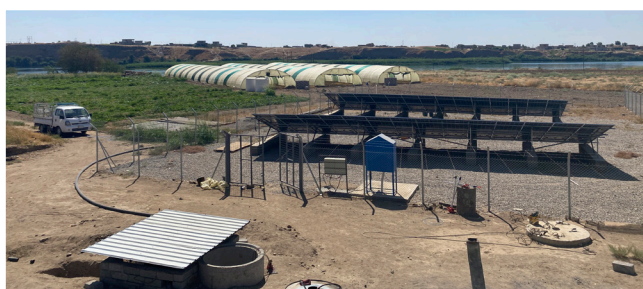
Green House and Solar System in Qavvarah
