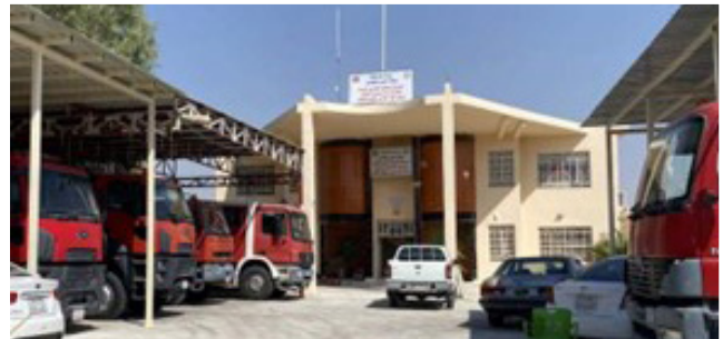
Hammam Al Alil Civil Defense Building, Ninewa
