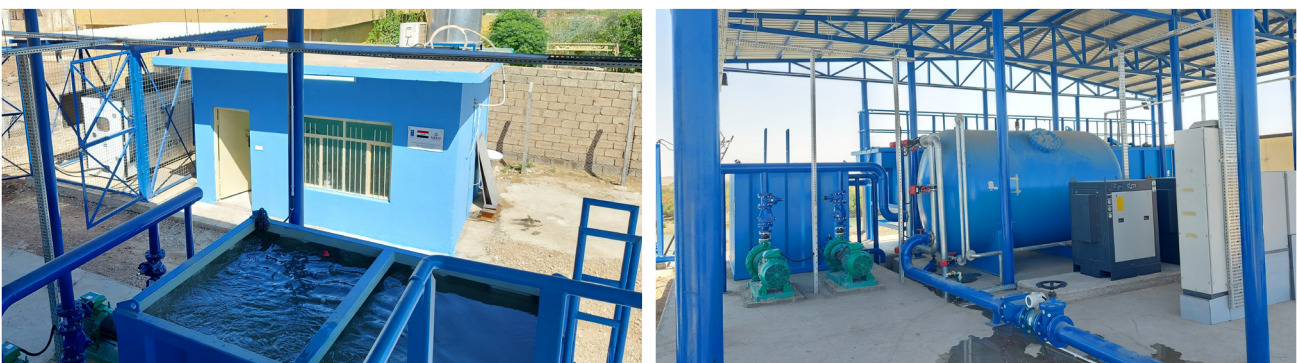
Rehabilitation of Al-Hasudiya Compact Unit, Namroud, Ninewa Governorate
