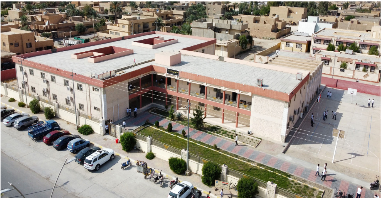
Rehabilitation of Rawa Secondary School for Boys, Rawa City, Anbar Governorate
