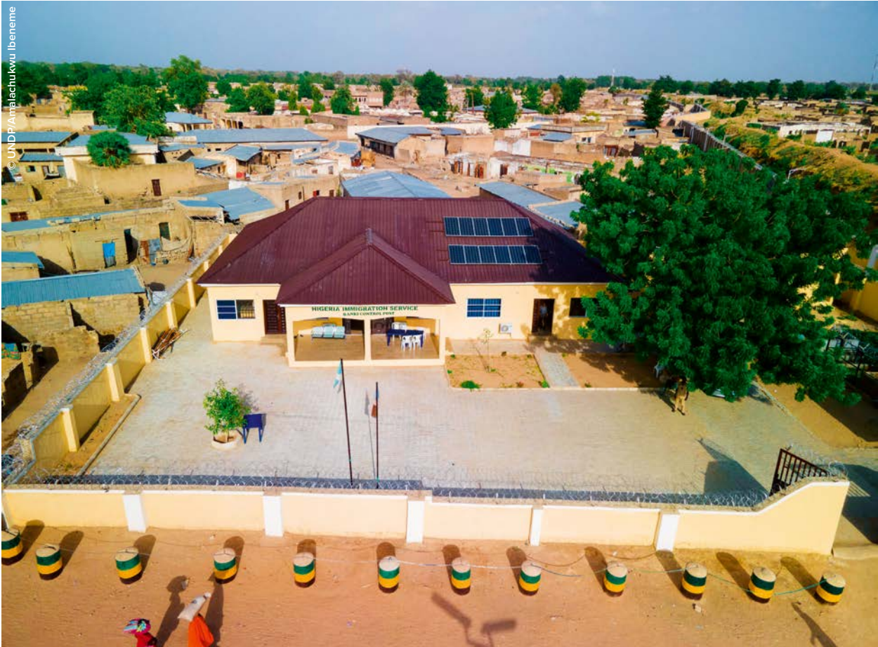
The newly-constructed immigration office in Banki will enhance cross-border commerce and security.
