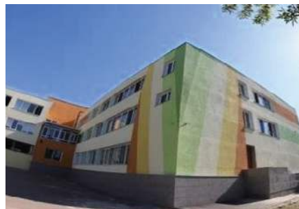
Picture 18. After reconstruction
