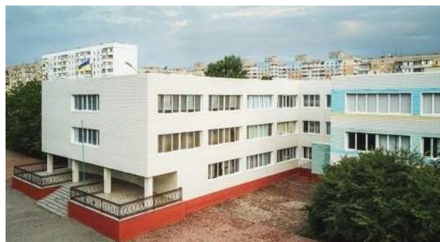
Picture 26. After reconstruction
