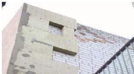
Picture 34. During reconstruction
