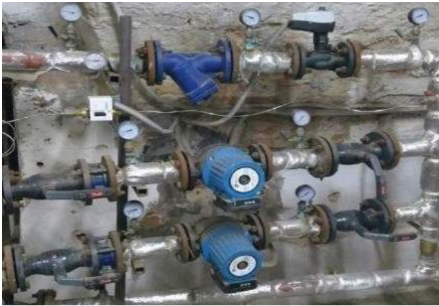
Picture 2. Heat carrier control nod
