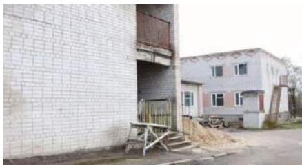
Picture 33. Before reconstruction
