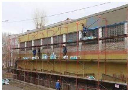
Picture 17. During reconstruction
