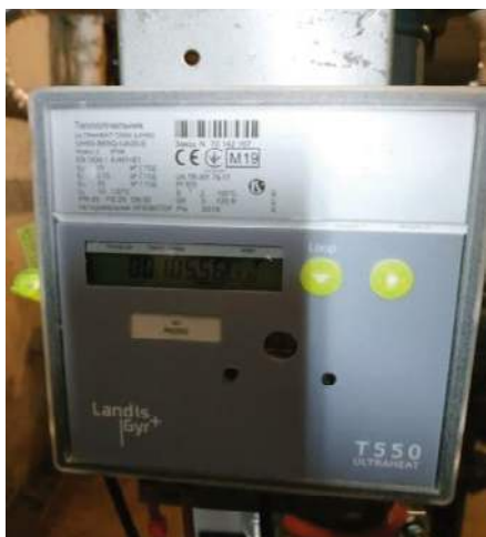
Picture 27. Heat meter Ultraheat
