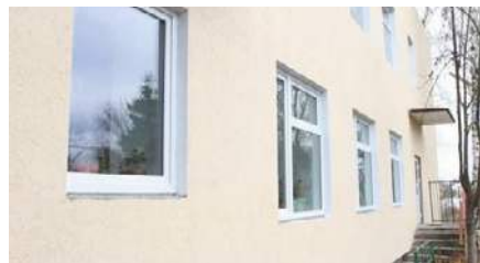
Picture 35. After reconstruction
