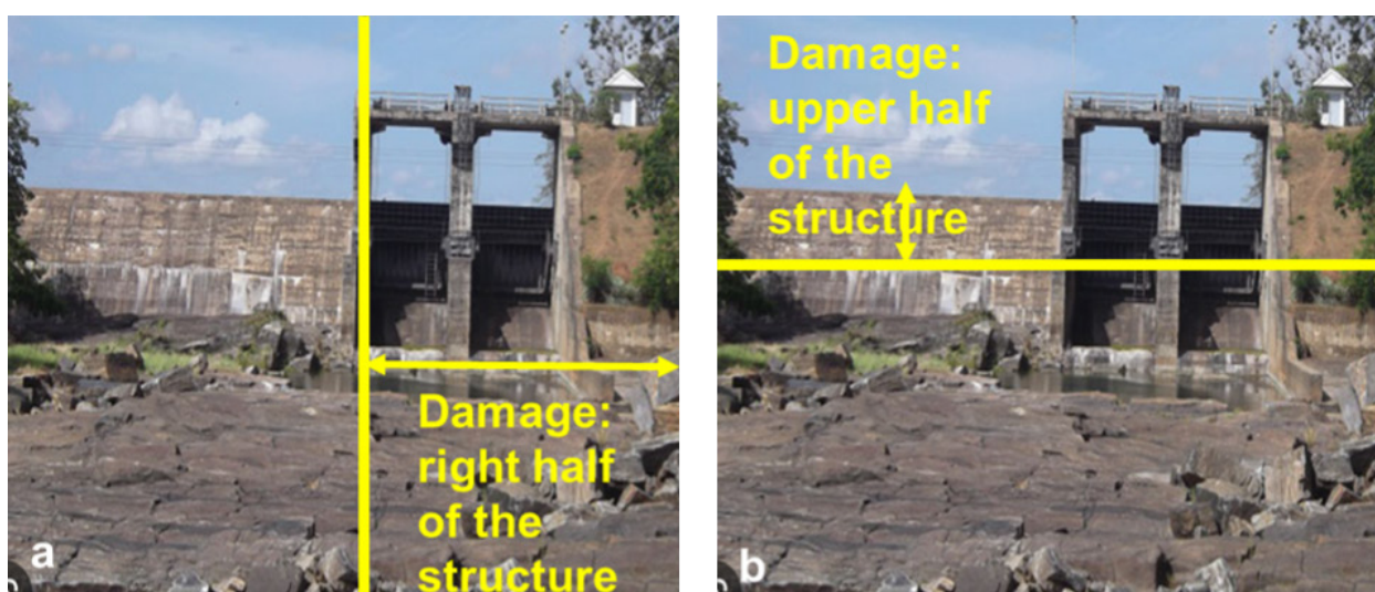
Figure 2.3 Damage assessment of partially destroyed irrigation structure
